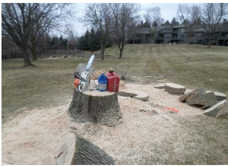
Removal of an ash tree that was not infested but severely decayed.
